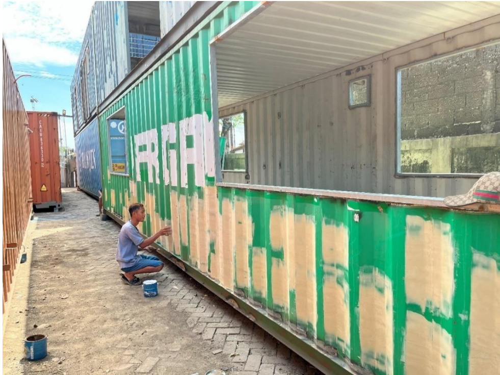
Lampiran 23 Gambar 4.2.1 Repair dan Repaint Kontainer
